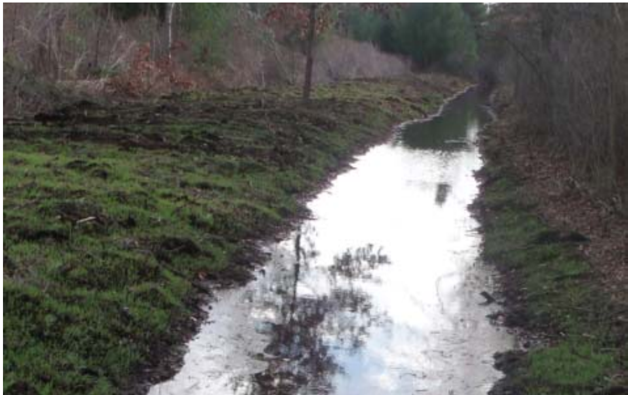
Orient-Fork Intercounty Drain
